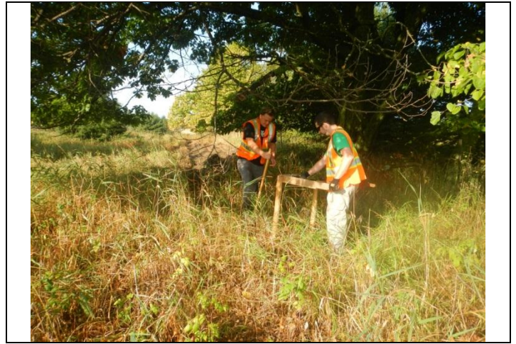
Photo 8 Excavating Test Pits Along Access Road From Lower 40 Foot Road To S28
