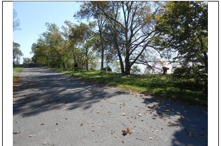
Photo 34 Excavating Test Pits Along Grass Strip Between Driveway and Lake Ontario
