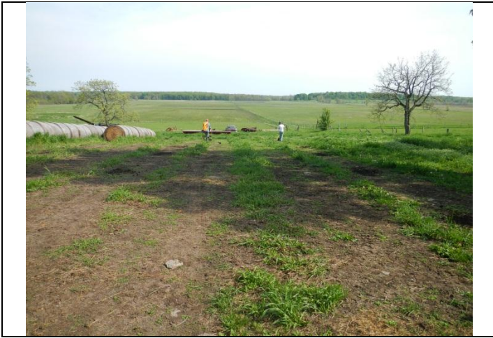
Photo 13 Excavating Test Pits Along Access Road, South of 2nd Concession, Looking South
