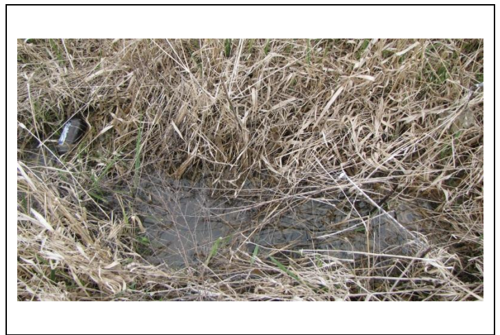
Photo 16 Standing Water in Turn Expansion, Dump Road
