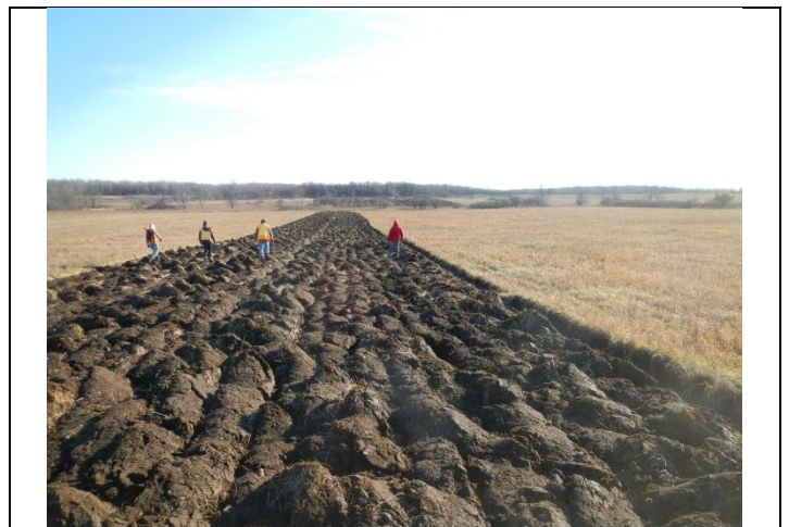
Photo 4 Surveying Access Road to S17, Looking South From 2nd Concession Road
