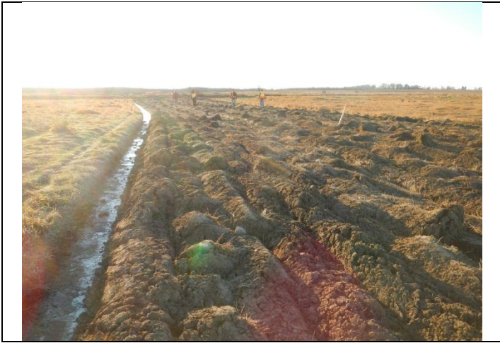
Photo 1 Starting Survey of Access Road to S15 and S24, From Front Road, Looking South.
